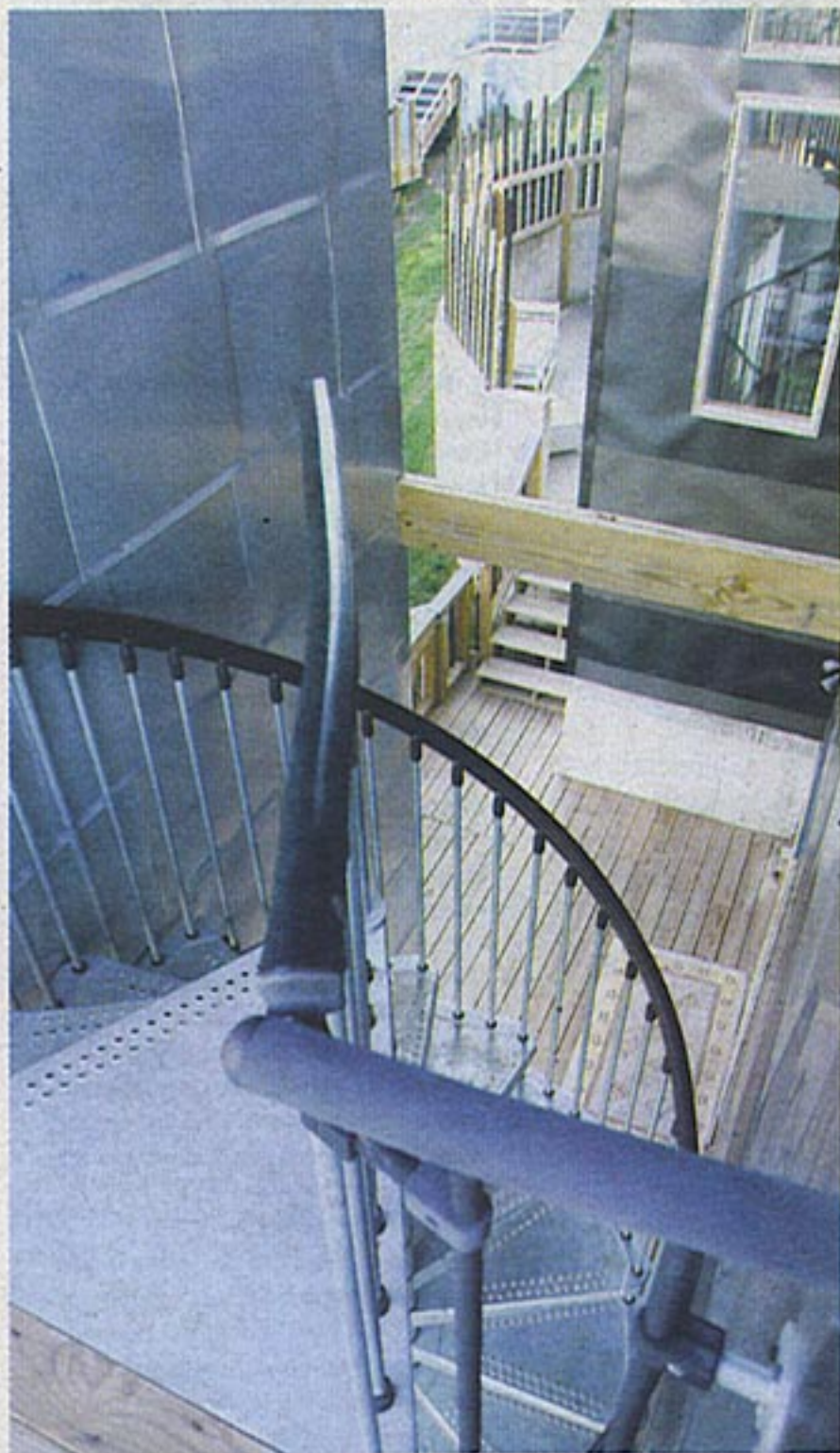
Spiral stairwells connect the upper and lower decks and the interior upstairs and downstairs.
